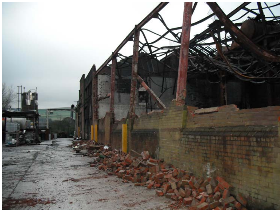
View of existing building
