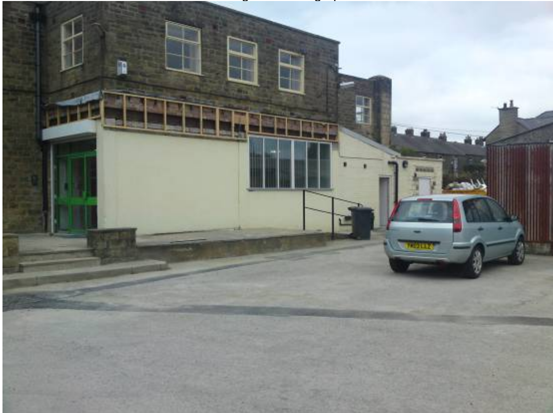
004 - Disabled access ramp to rear of property. DDA/ DOC M compliant handrails to be installed.
