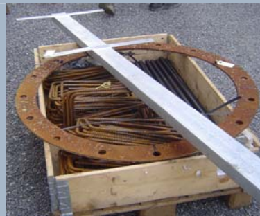
Control Cabinet Stand, Bolt Circle Template, & U-Braces
