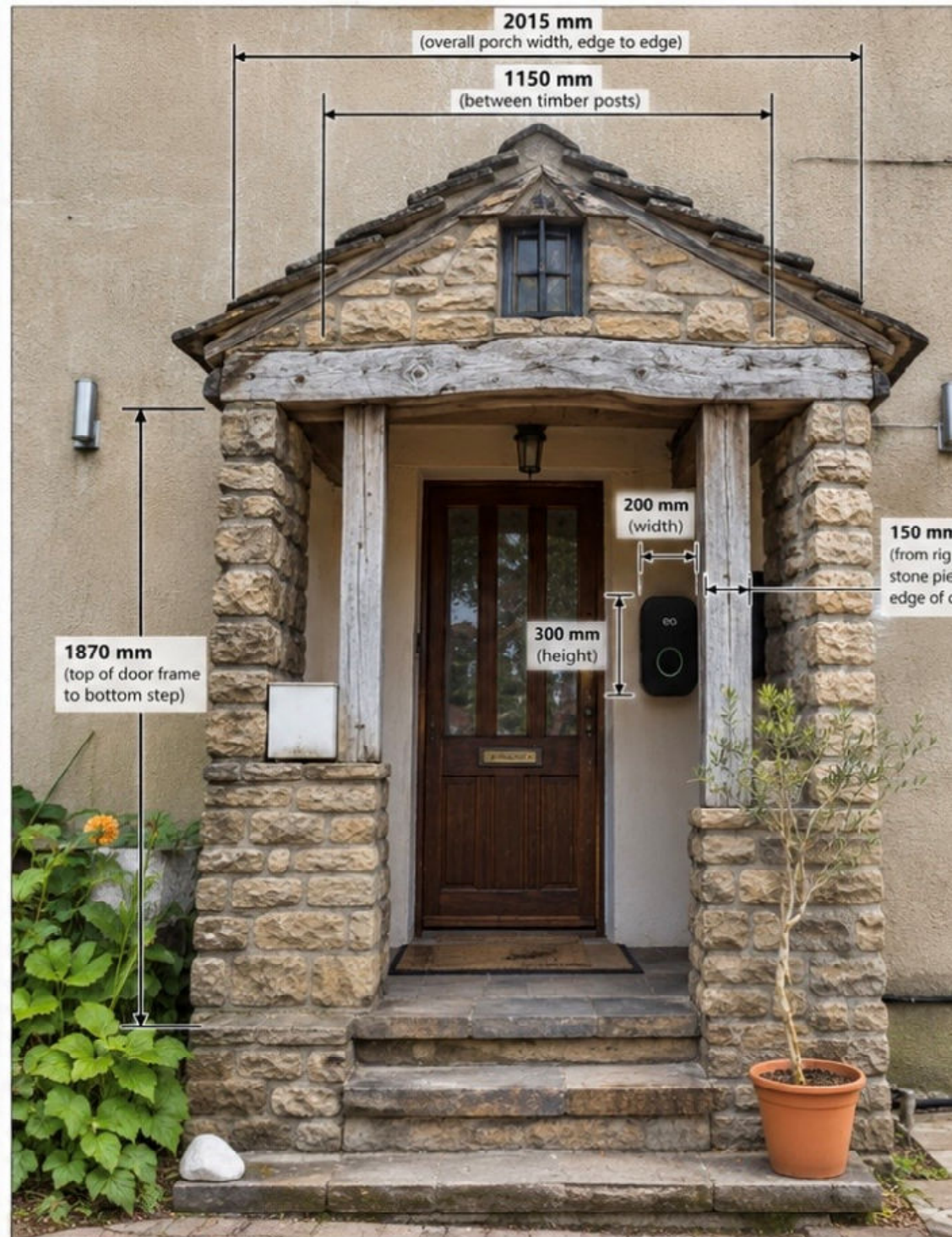
02 PROPOSED PORCH (FRONT VIEW WITH EV CHARGER)
