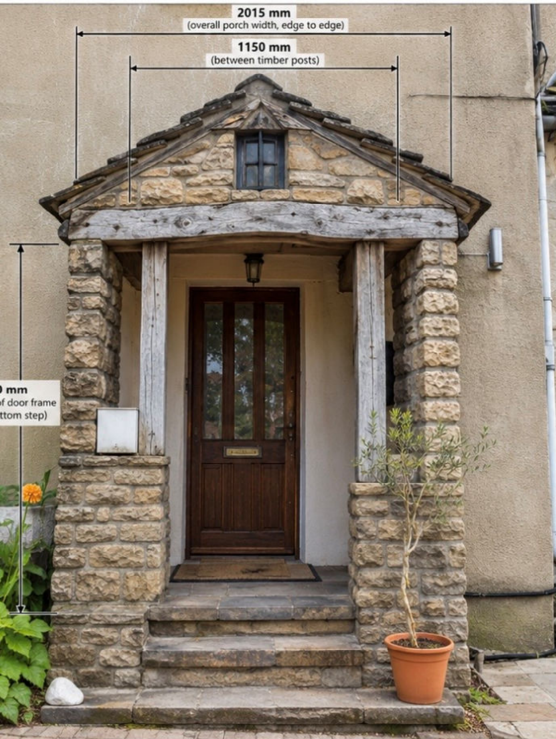
EXISTING PORCH (FRONT VIEW)
