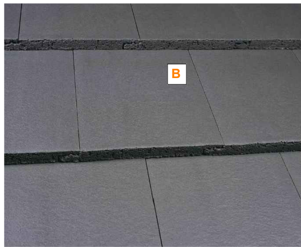
B – INTERLOCKING ROOF TILE
