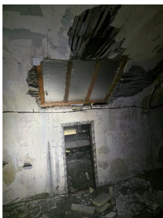
Image 11: Crawl space view with Kingspan present
