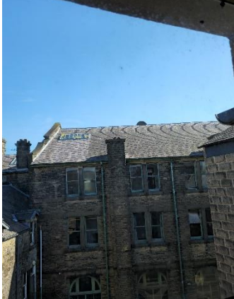
Image 16: Area below the upper dwelling space.
