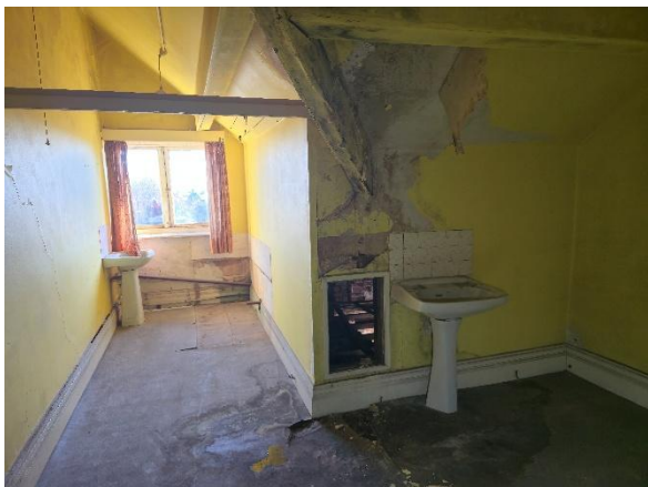
Image 7: Indication of one of three small crawl spaces on the western aspect of Hardwick Hall
