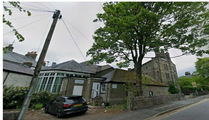
Figure 7 View to Rear of Site along Hardwick Square South
