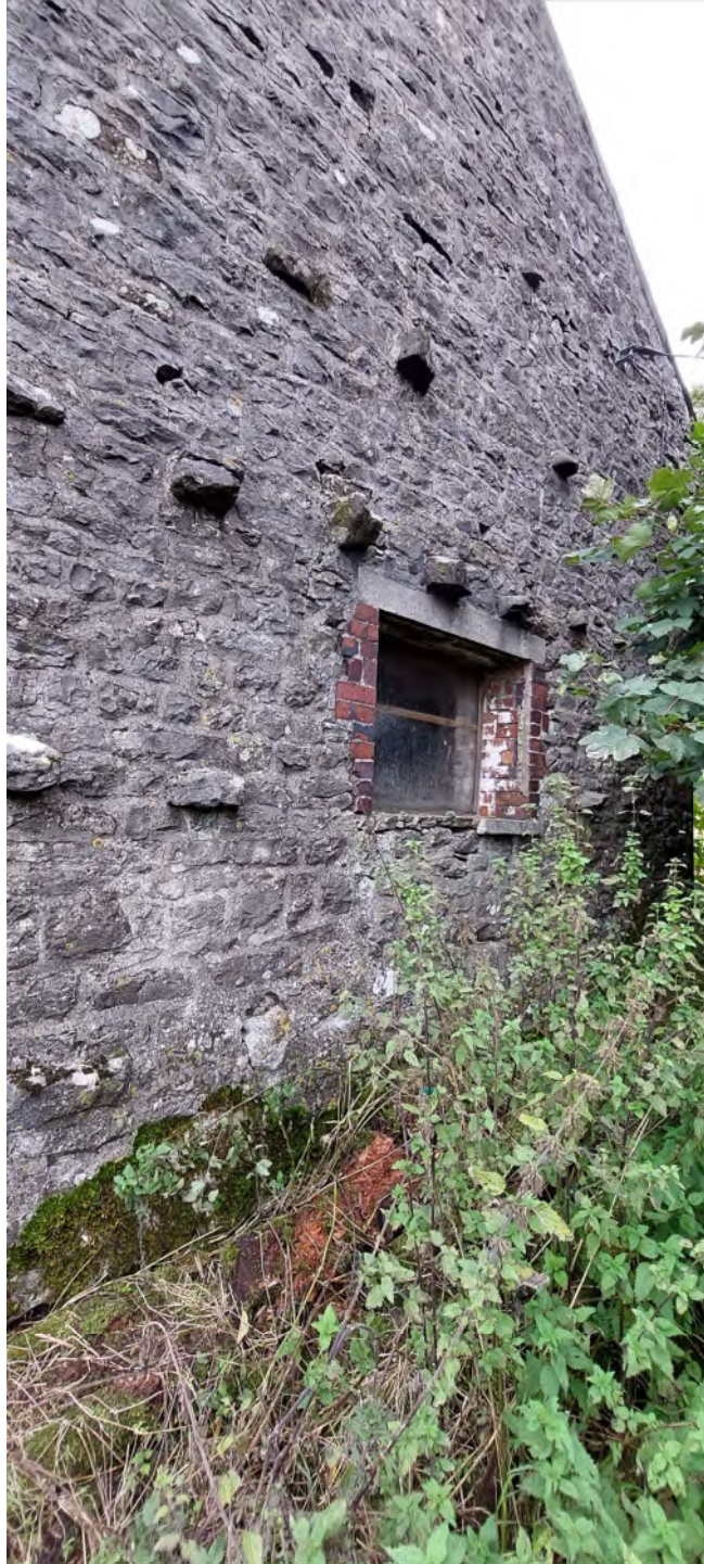
Picture3- Replacement of stonework with brick work on either side of window at the east elevation (Gable wall).
