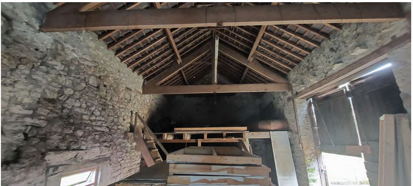
Picture5- A first floor had been installed within a small portion of the building at the west side.
