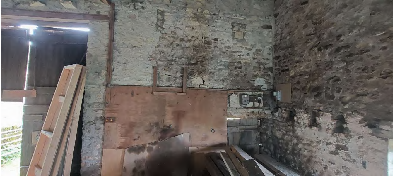
Picture4- The electrical meter is positioned on the east side and is visible from the inside on the north wall.
