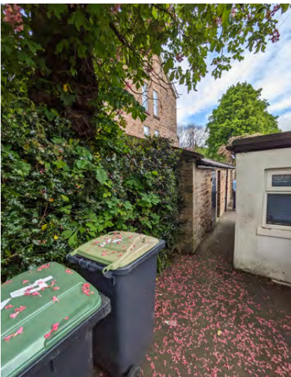
Figure 4 Rear of Unit 1 from Cresswell Street
