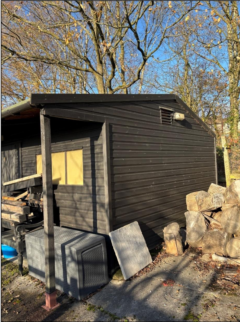
Photograph 1. End of B1.
