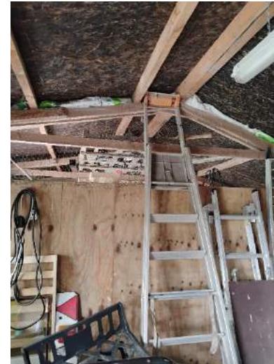
6. Chicken wire installed across roof timbers.
