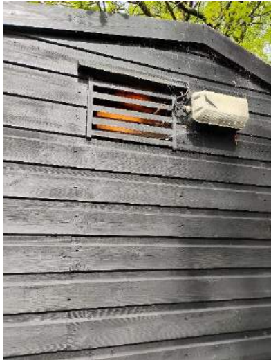
4. Louvered vent on east gable.
