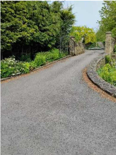
10. Driveway leading to site from Lower Hague.
