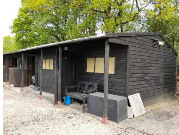
2. South elevation and east gable.
