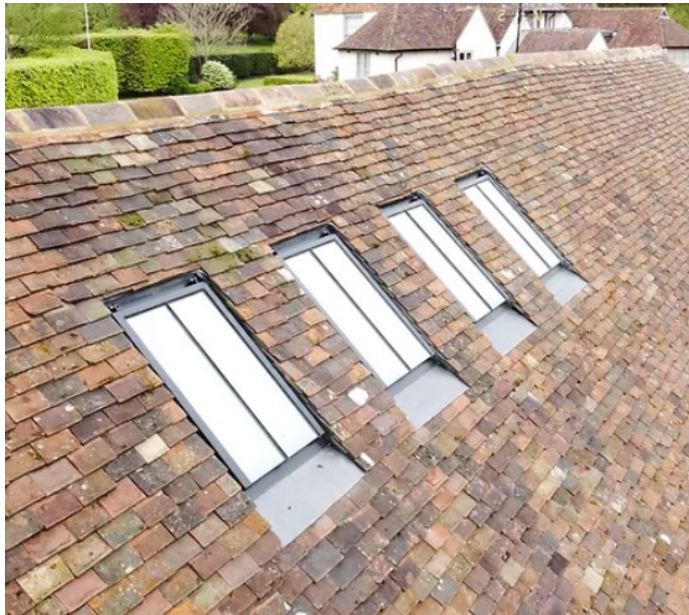
STELLA CONSERVATION ROOF LIGHT AS INSTALLED
