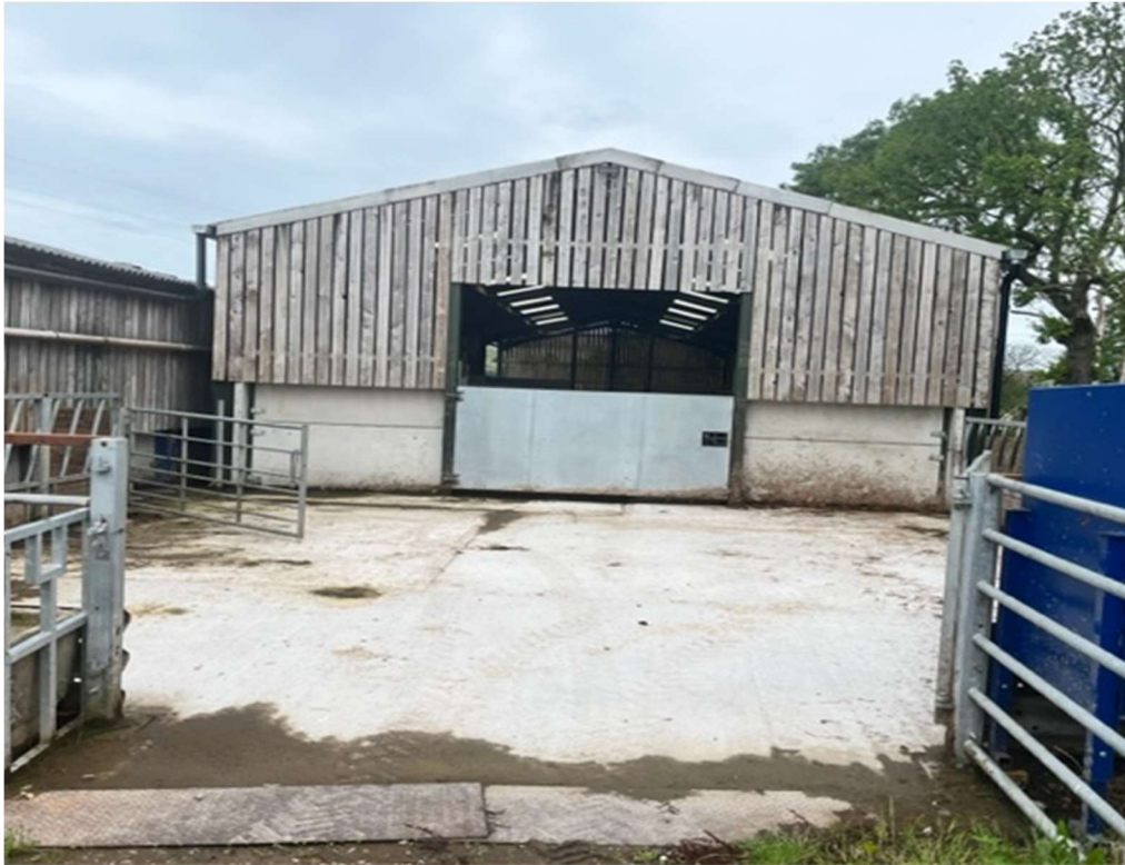
Photograph 1: Location of feed yard for the proposed roofing over.
