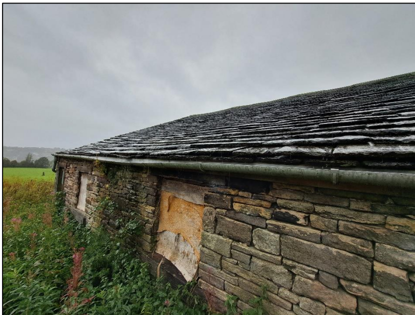
Photograph 3 showing the roof
