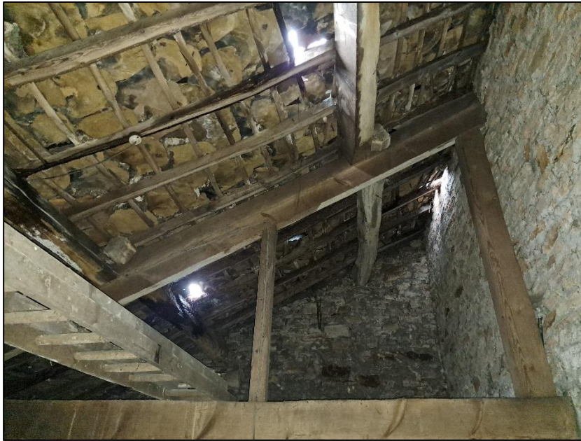
Photograph 6 showing the internal roof structure
