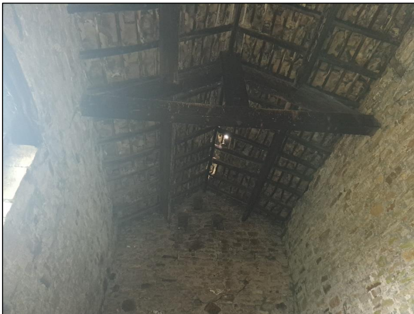
Photograph 5 showing the interior of the building
