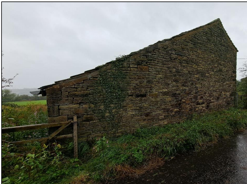
Photograph 1 showing the building
