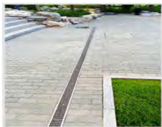
Figure 18 – 19. Oil Interceptor - Trapped linear drainage channels.
