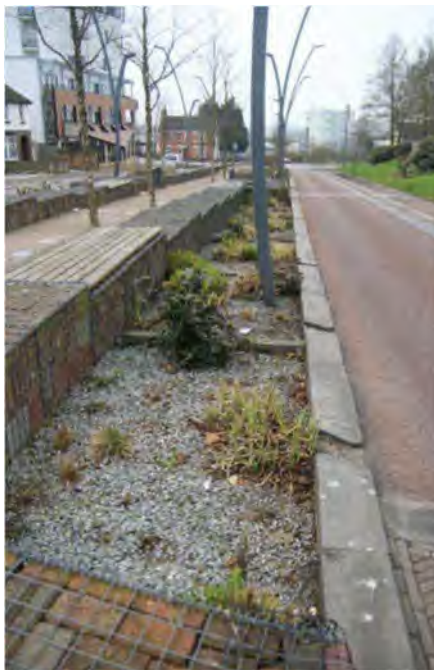
Figures 21 & 22. Bioretention Area & Rain Garden
