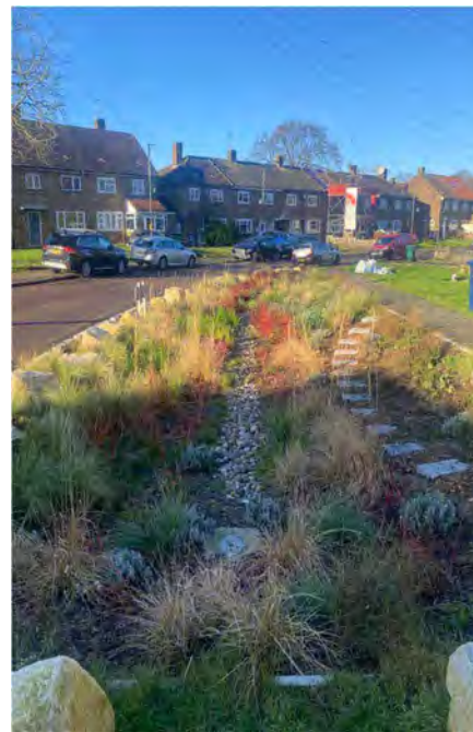
Figures 21 & 22. Bioretention Area & Rain Garden
