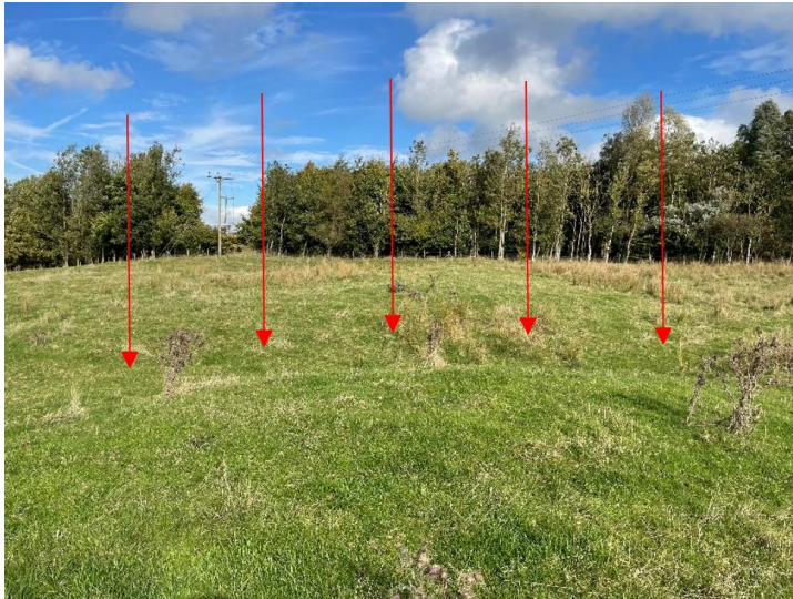
Plate 4: Proposed crossing point showing quarrying scarring (red arrows) 3.5m wide
