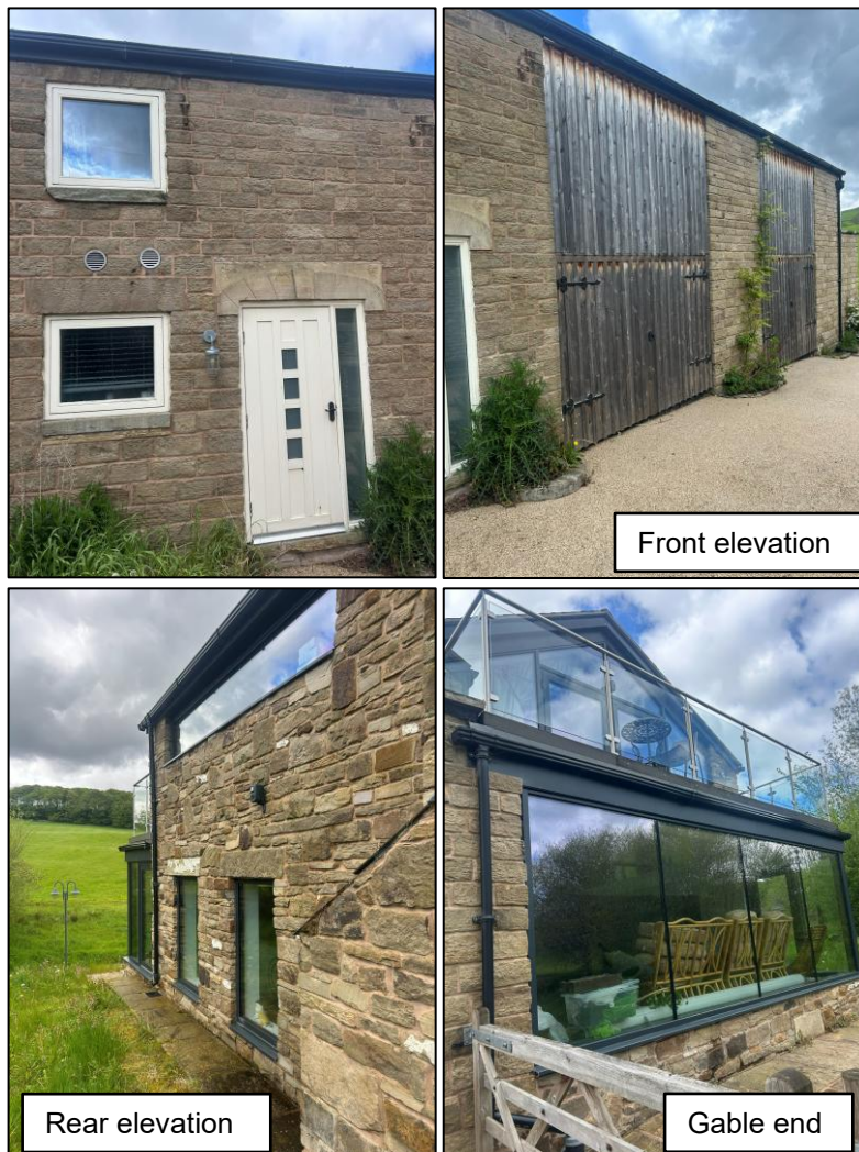
Figure 4.1 - Photographs of front, rear and gable elevations
