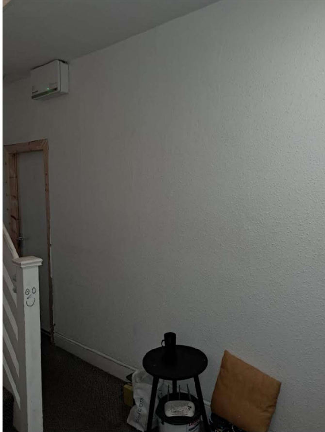
Figure 2 - Wall to be removed bedroom area
