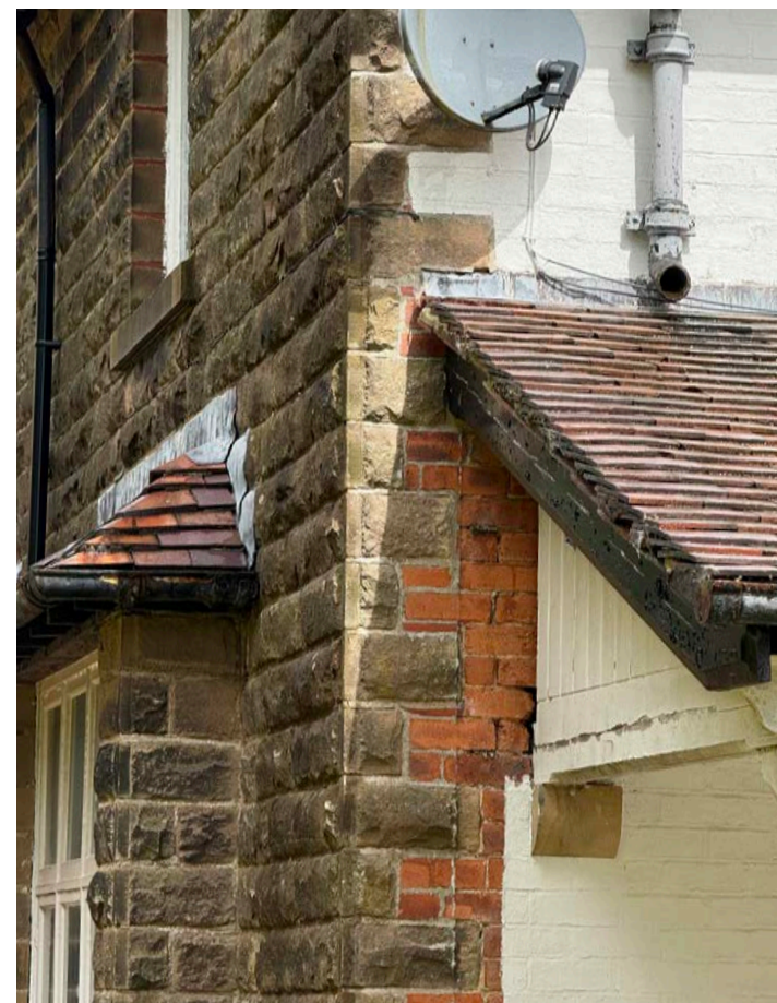
Detail of existing veranda
