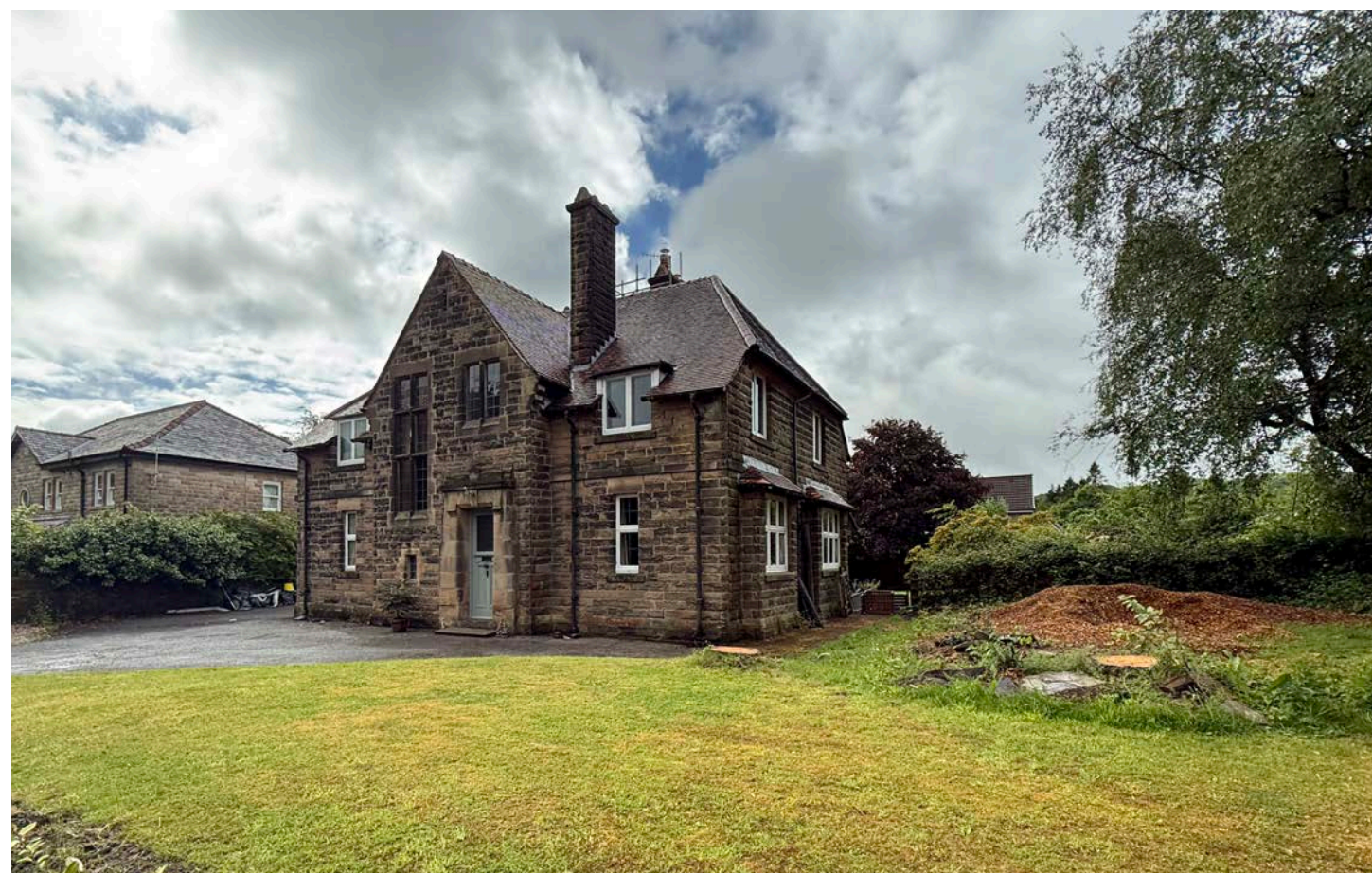
Corner between Front Elevation and West Elevation
