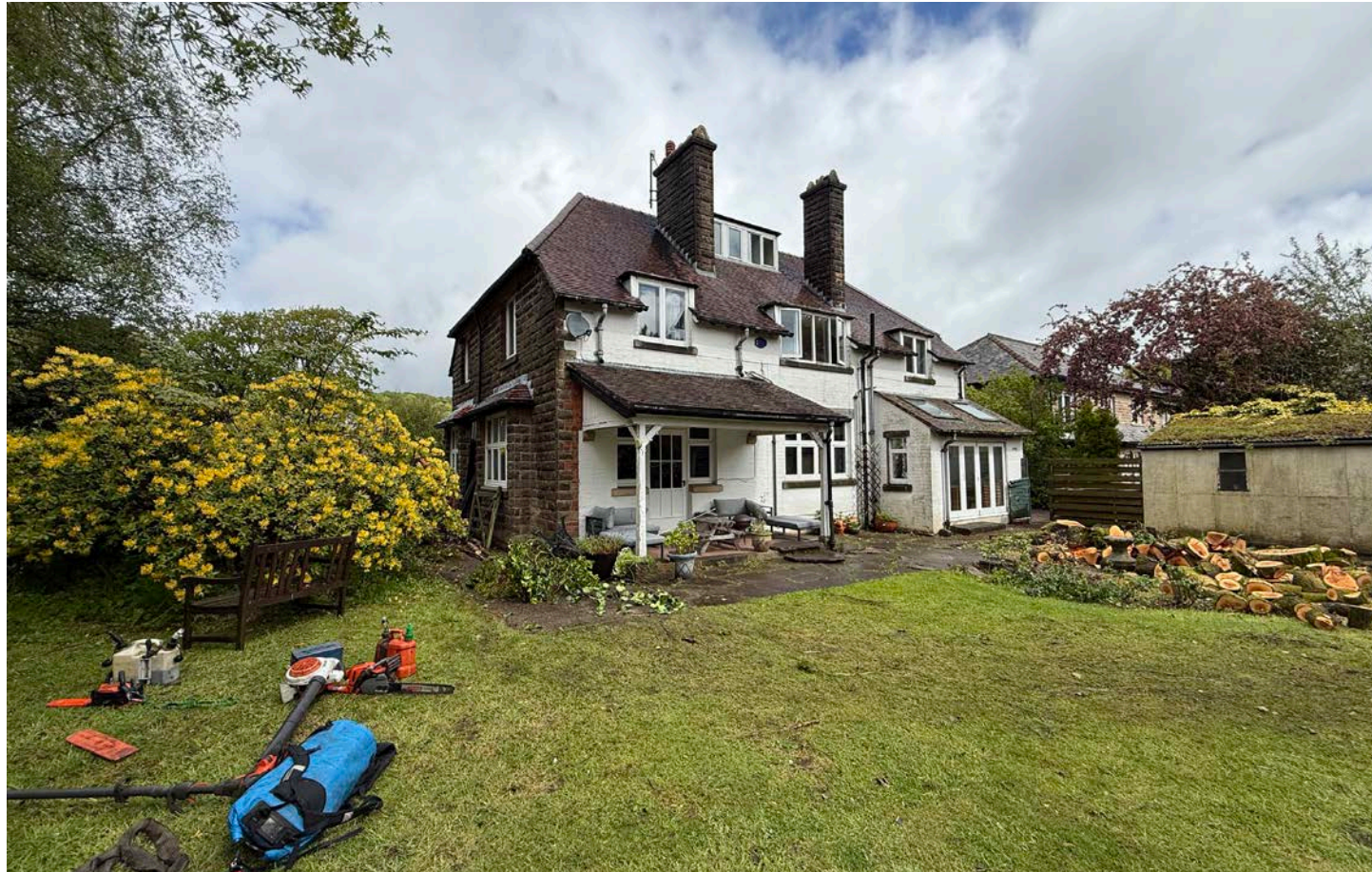
Front Elevation from SW corner
