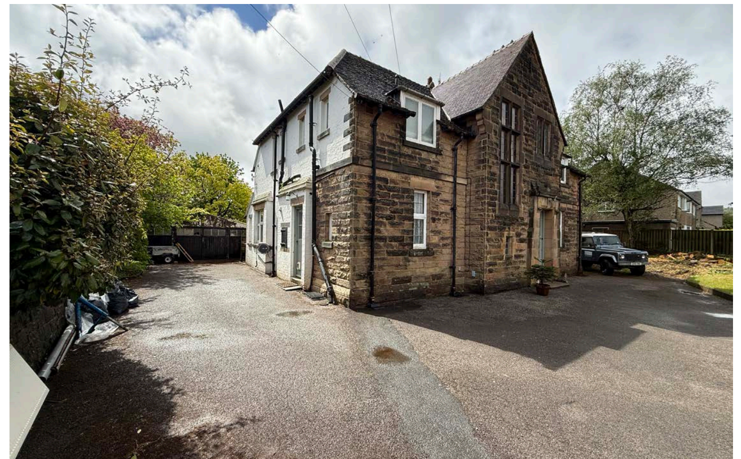
Corner between Front Elevation and East Elevation
