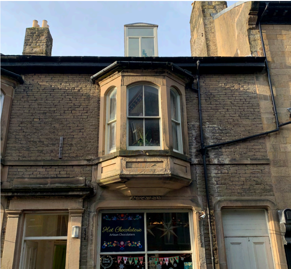
string courses at first floor level
