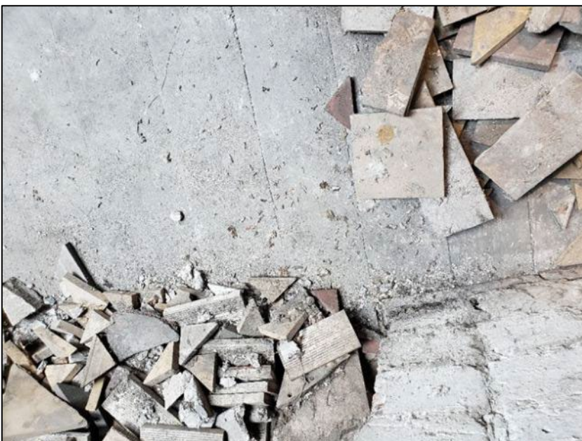
Photograph 15 Showing an accumulation of bat droppings beneath the apex within the eastern gable void
