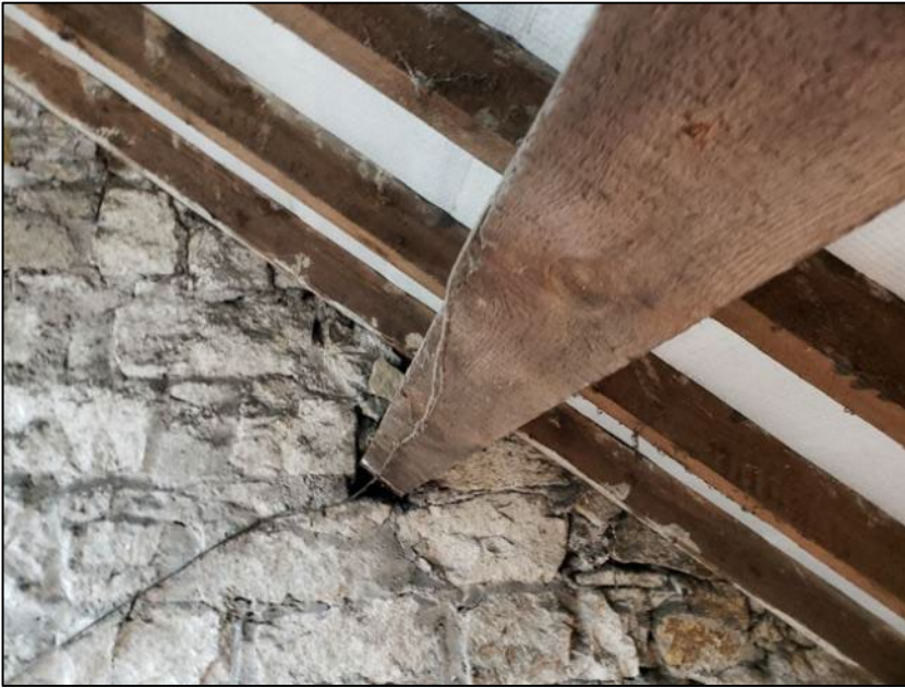
Photograph 13 Showing the potential access point around the roof purlin on the eastern gable
