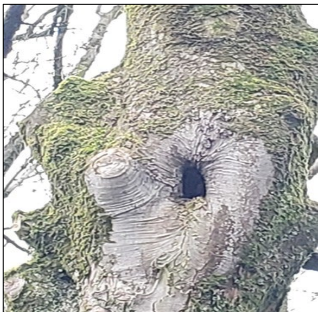
Photograph 25 Close up of Tree T27 with a knot hole leading to a cavity (PRF-M)
