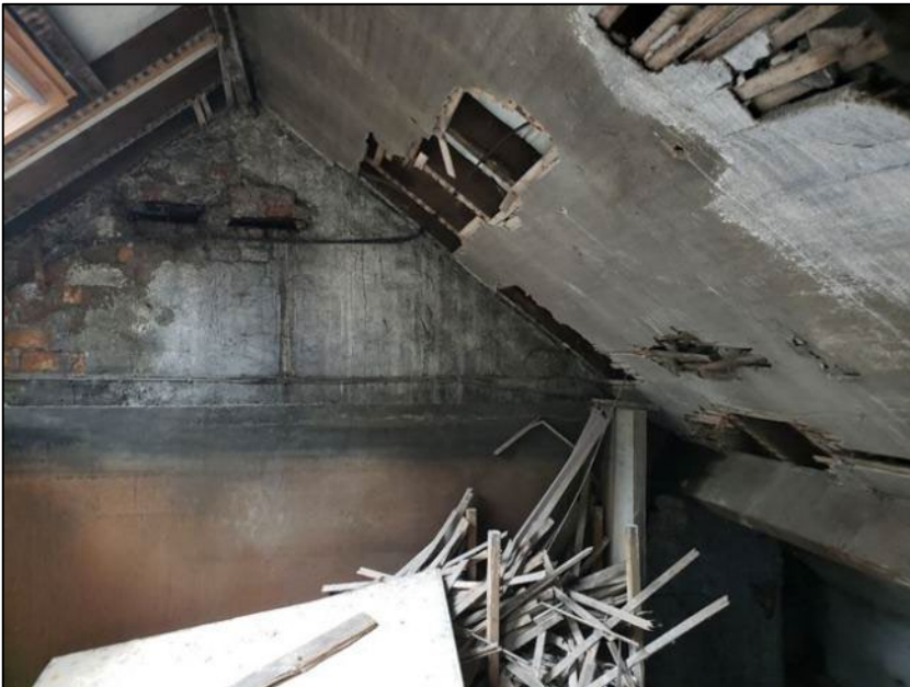
Photograph 17 Showing the section of roof void where lining is partially dismantled within the western gable void
