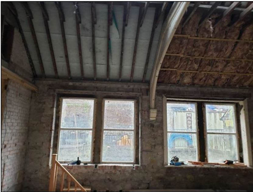
Photograph 10 Showing the exposed masonry and exposed roof lining and insulation of the first floor
