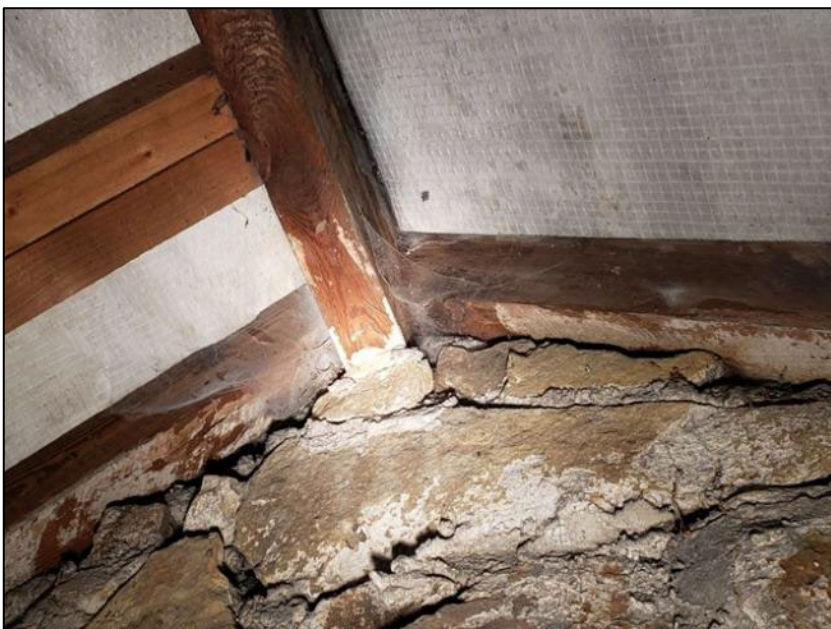
Photograph 12 Showing the potential access point at the interior of the eastern gable apex
