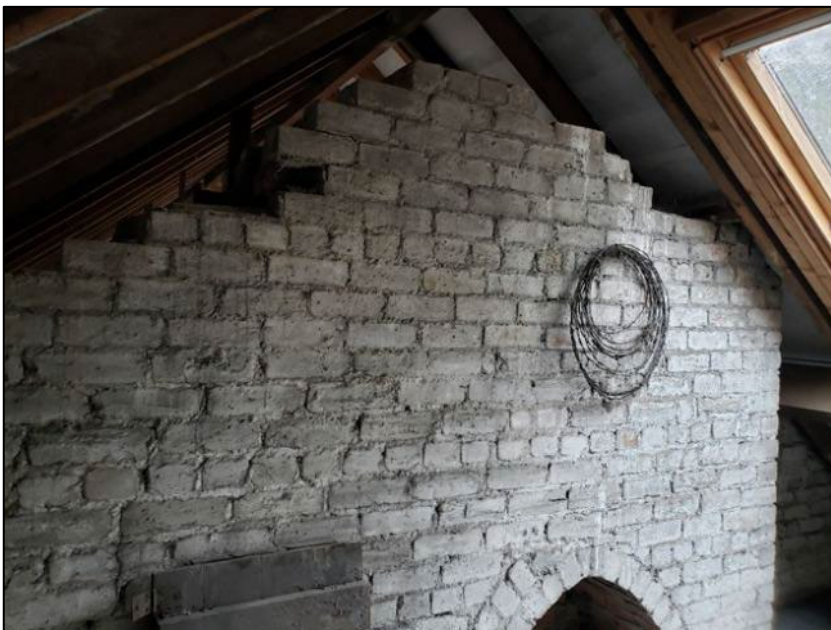
Photograph 11 Showing the open void above the eastern rooms allowing access from the void into the rest of the first floor rooms
