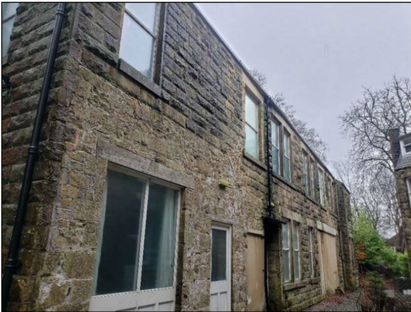
Photograph 1 The Coach House southern elevation
