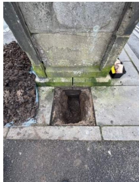
Photo 2 – Trial pit to north side of cistern
