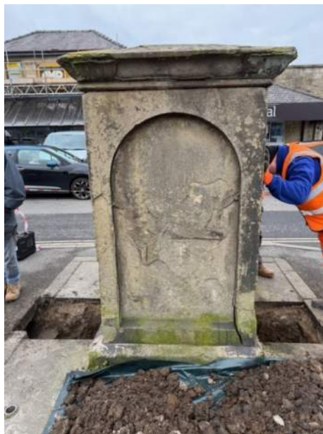
Photo 1 – East elevation of cistern
