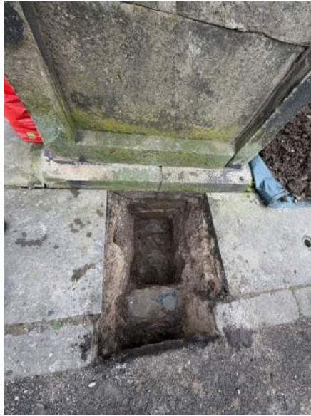
Photo 3 - Trial pit to south side of cistern
