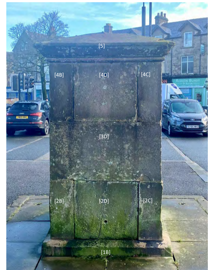
West Facade Existing Photograph (nts)
