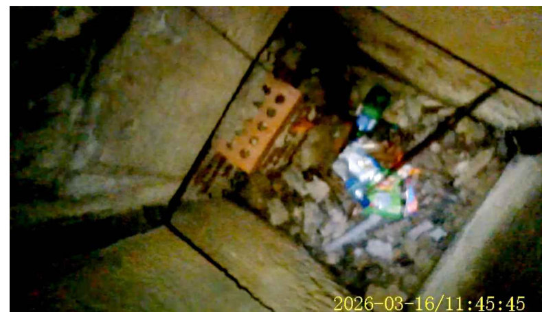
06. Interior view showing 20th/21st century engineering brick to rear of lower tap-hole panel.
