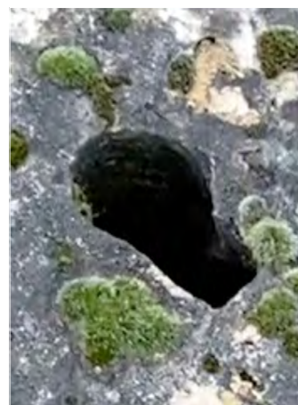
05. Detail of pedestal fixing aperture.
