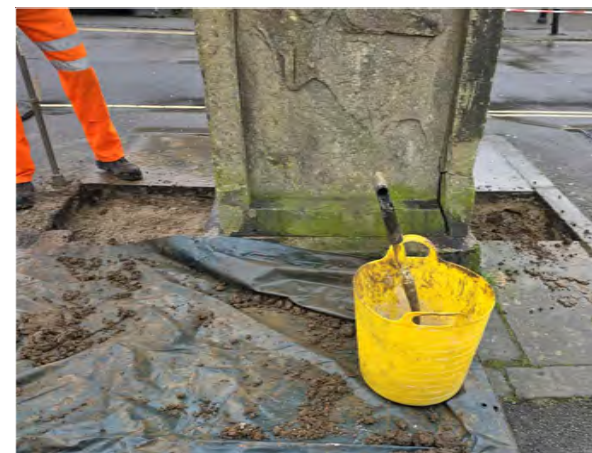
01. Opening up works in progress below paving to south and north elevations.
