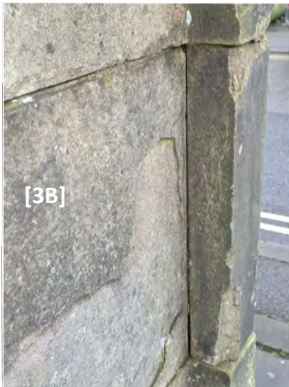
Extent of surface loss to central panel [3B]
