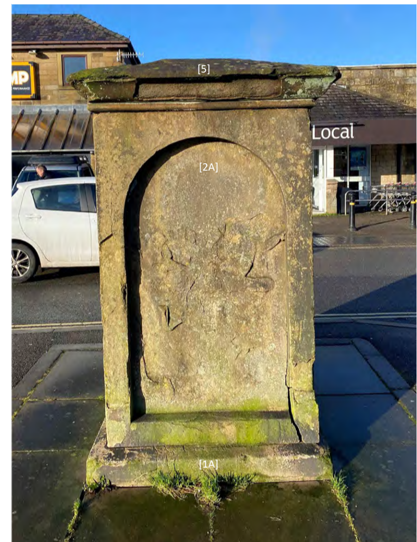
West Facade Existing Photograph (nts)
