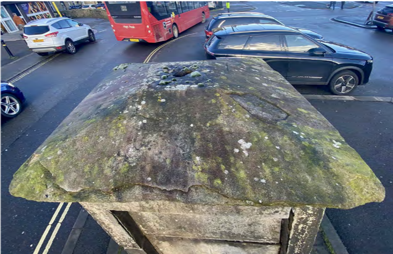
Cornice [5] South Top View
