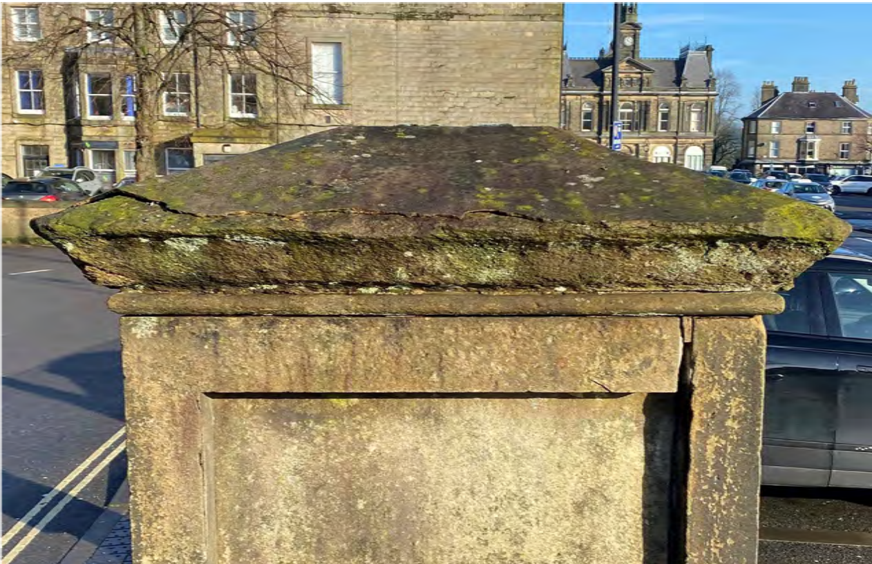
Cornice [5] South Elevation View
