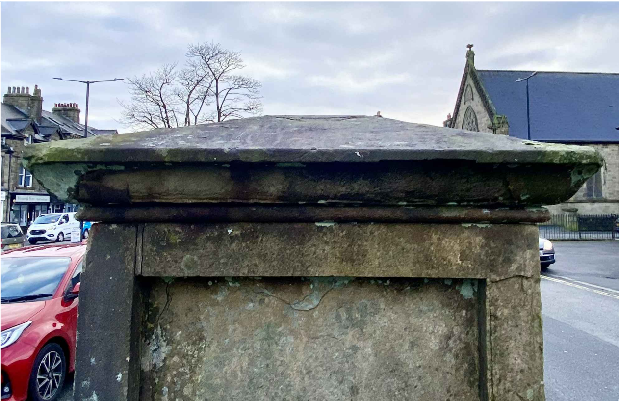
Cornice [5] North Elevation View
