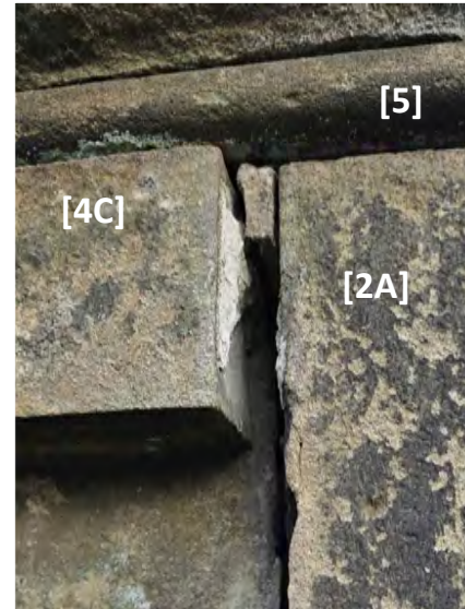
(above & above right) Portland Cement pointing (D1 Defect) to fill structural displacement gaps >10mm between east facade Cavendish panel [2A] and panel [4C]. Severe surface deterioration >10mm spalling (Type C1 defect) to southeast corner of Cornice [5].
