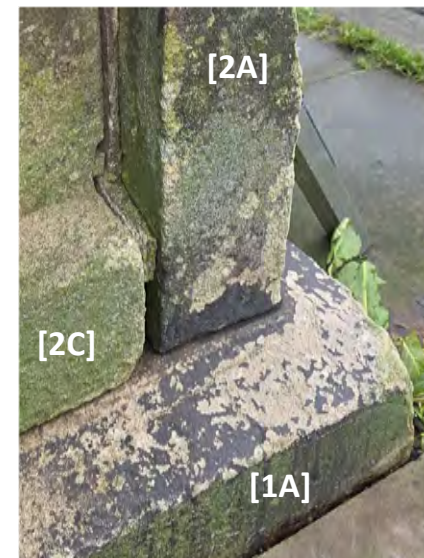
Portland Cement (D1 Defect) to fill structural displacement gaps >10mm at southeast corner [2C] [2A] & Plinth [1A]
