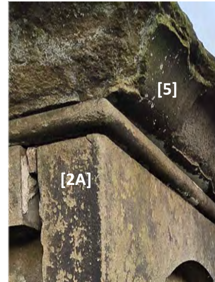
(above & above right) Portland Cement pointing (D1 Defect) to fill structural displacement gaps >10mm between east facade Cavendish panel [2A] and panel [4C]. Severe surface deterioration >10mm spalling (Type C1 defect) to southeast corner of Cornice [5].
