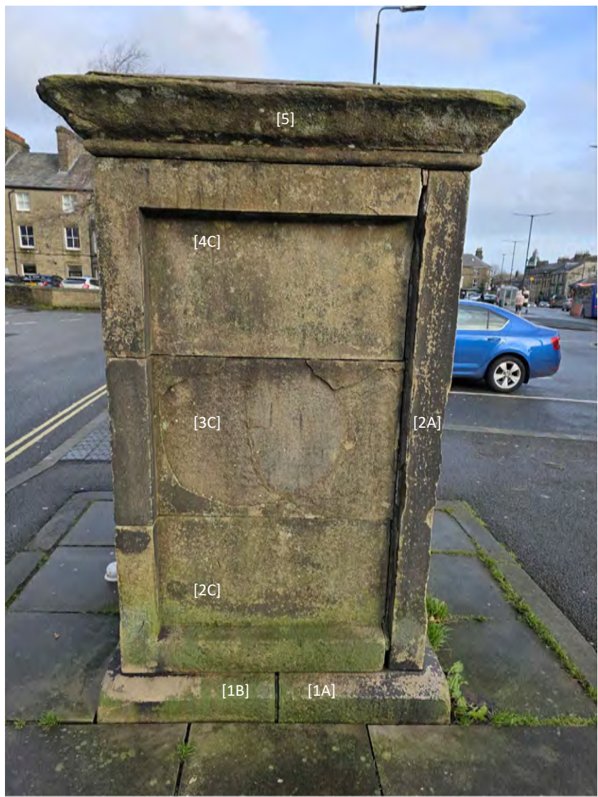
South Facade Existing Photograph (nts)
