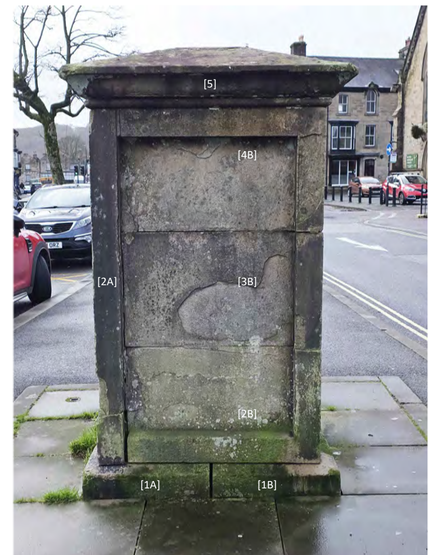
North Facade Existing Photograph (nts)
