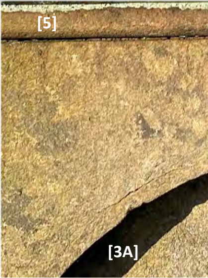
(above & above right) Cracking <10mm (Type B defect) to Cavendish Motif frame and above arch section [2A] and Severe surface deterioration >10mm spalling (Type C1 defect)
