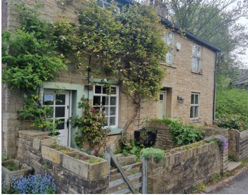
Figure 3: Chartwell Green window frames to 2 and 4 Wellgate, opposite Wesley House at the junction of Wellgate, Wesley Street and Hope Street.
