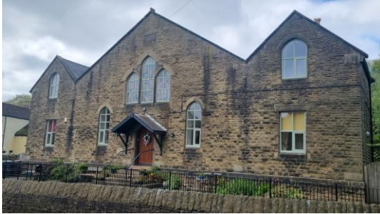
Figure 4: Chartwell Green window frames to the former Wesleyan School, opposite Wesley House across the stream.
