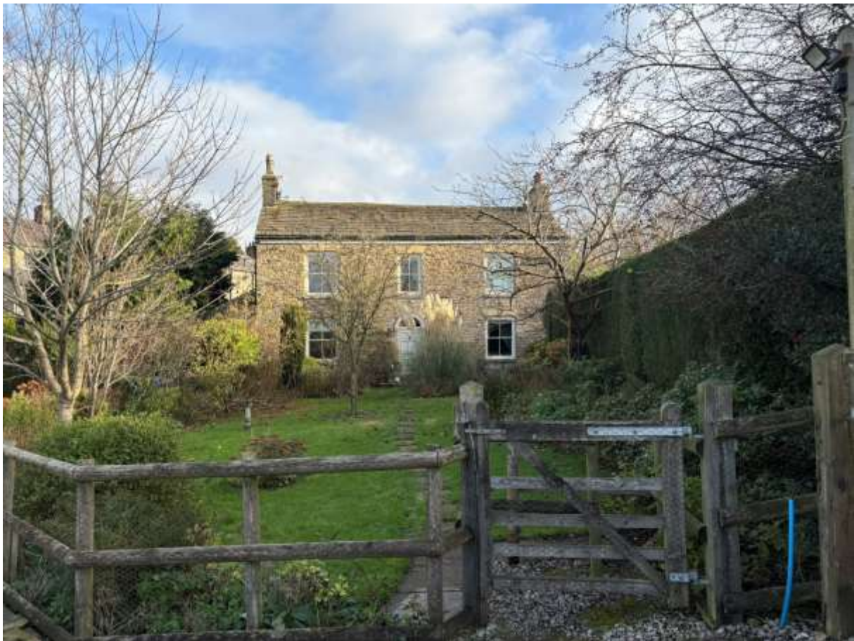
Image 1. The farmhouse now sits within its own domestic curtilage with a gate and pathway leading from the west. The principal elevation faces away from the road which reflects the building's historic function and setting.
