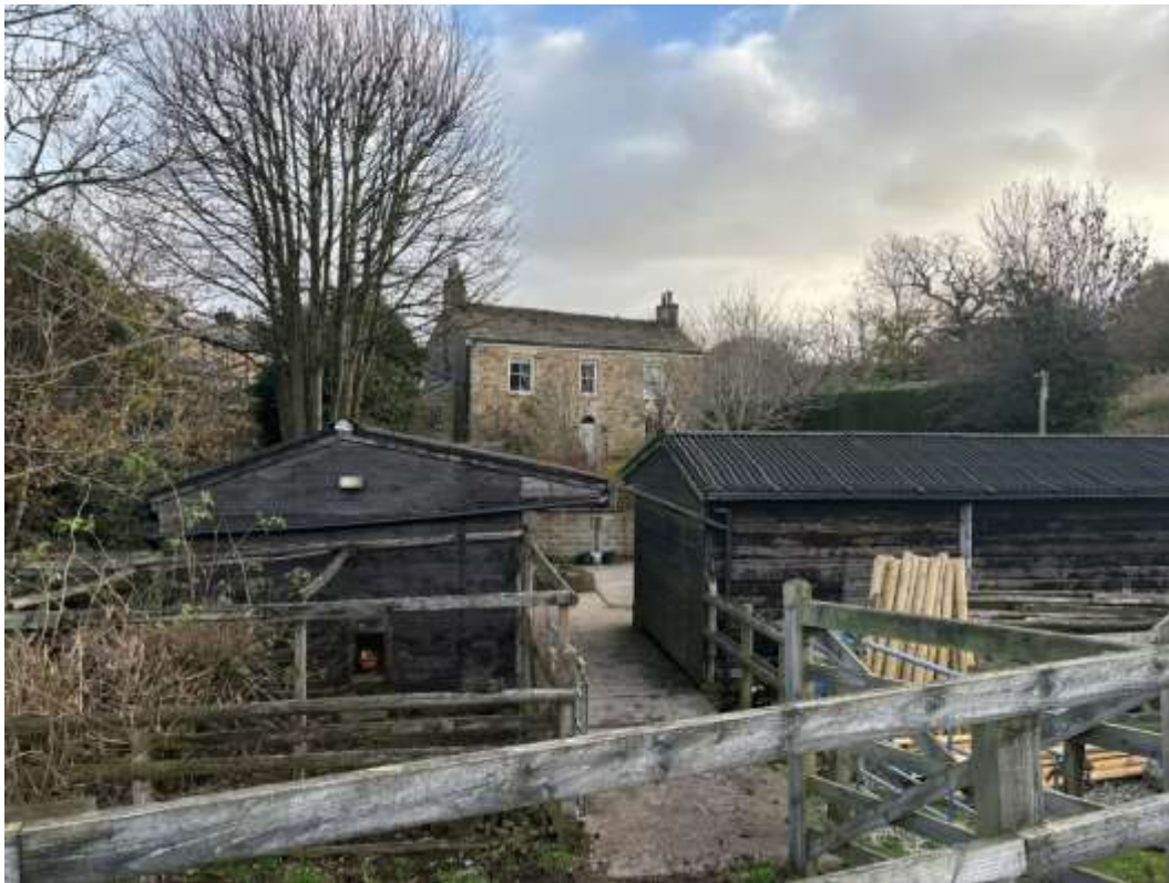
Image 5. The existing modern stables restrict views through to the principal elevation of the farmhouse. Historic views such as this contribute to the setting of the building and the removal of the stables will offer some minor benefit as a consequence of the proposals.
