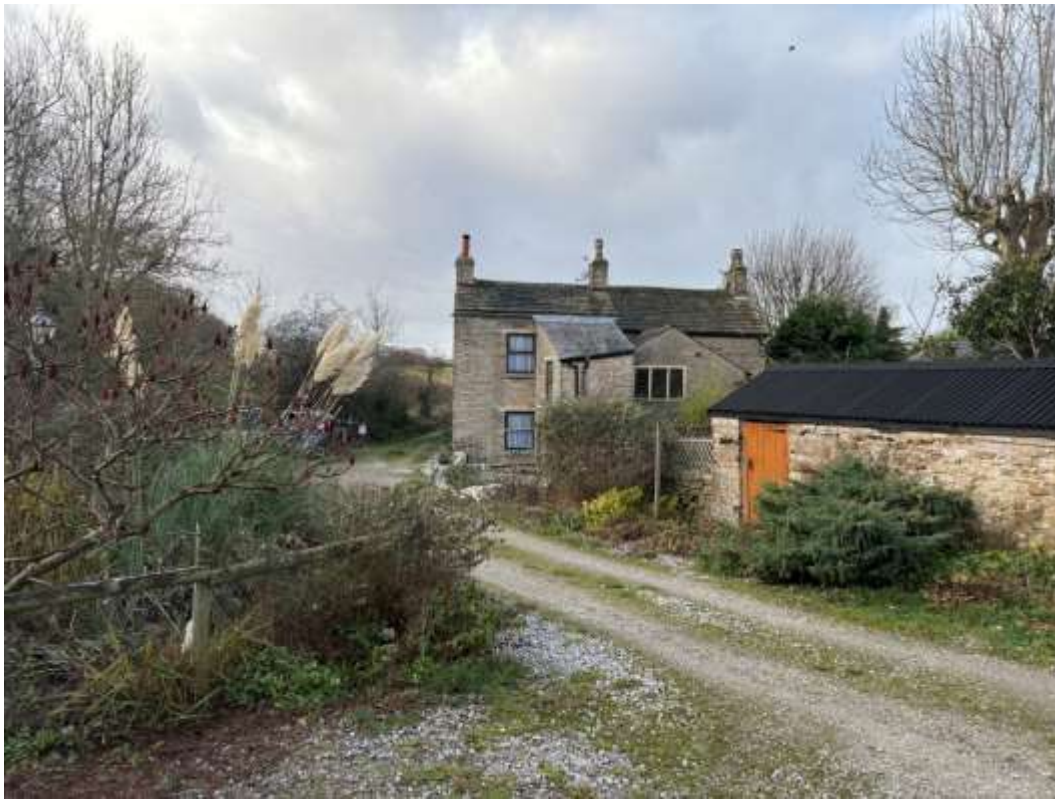
Image 2. The development site cannot be seen from the main road. In terms of impact, this primarily relates to the setting of the building as viewed from the west towards its principal elevation.
