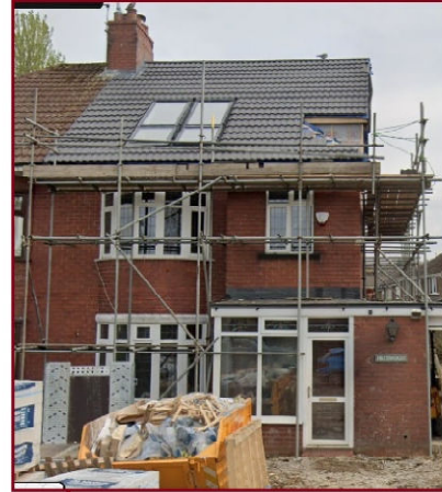
HILLSWOOD, SIMMONDLEY LANE: Red brick finish, white and anthracite UPVC windows, large wood clad dormer (when finished)
