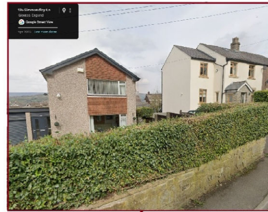
139(L), SIMMONDLEY LANE: Pebble dash and clay tile finish, anthracite PVC cladding, white and anthracite UPVC windows / fascias
