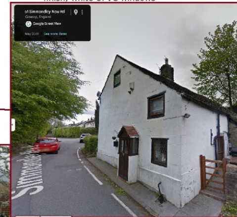
51, SIMMONDLEY NEW ROAD: White painted block finish, walnut UPVC windows
