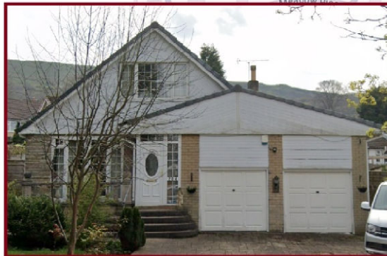
SUBJECT PROPERTY: 204, SIMMONDLEY LANE Current finishes: White PVC cladding, yellow brick, white UPVC windows
