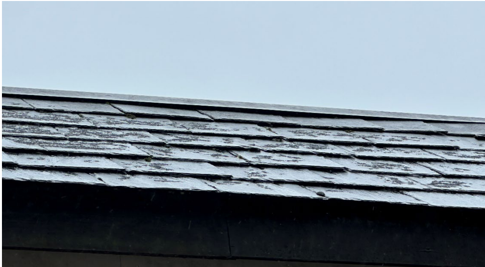
Photo 4: Tiles are generally tight fitting, small gaps along the capping provide PRFs.
