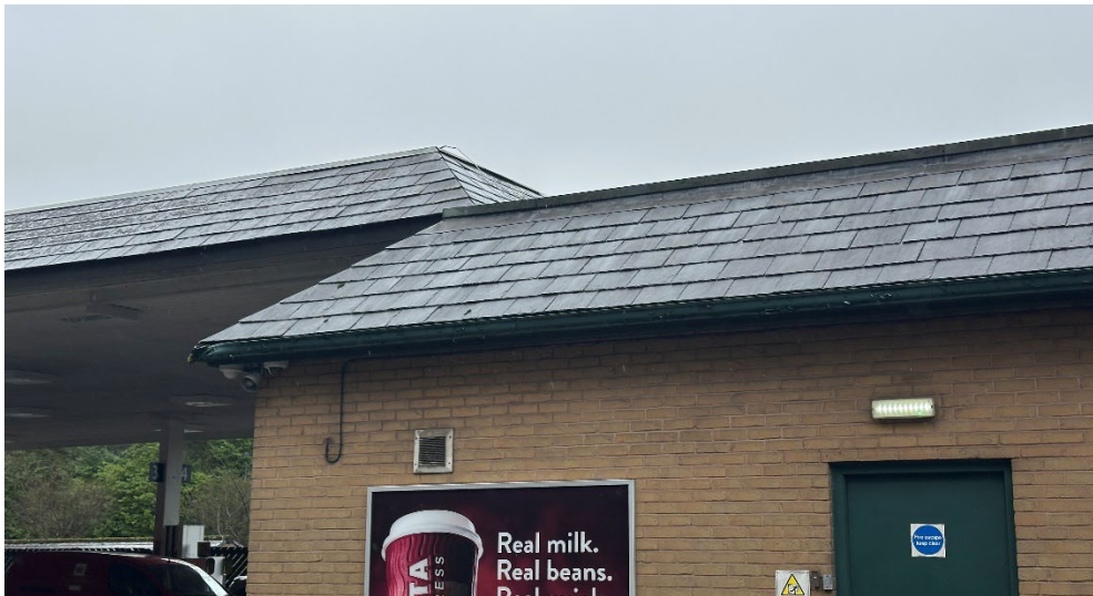
Photo 2: Slates are intact with no apparent lifted or slipped tiles.
