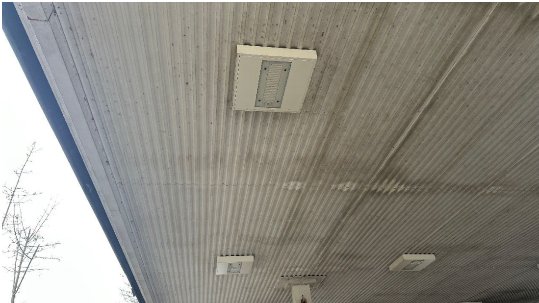
Photo 7: The canopy cover is entirely sealed and in good condition.
