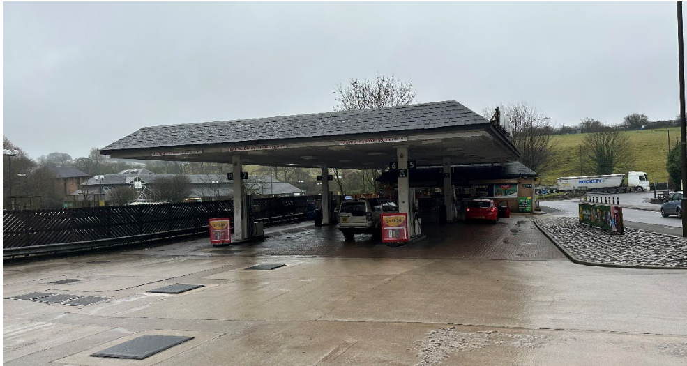
Photo 1: The Site consists entirely of hardstanding, with no vegetation present.
