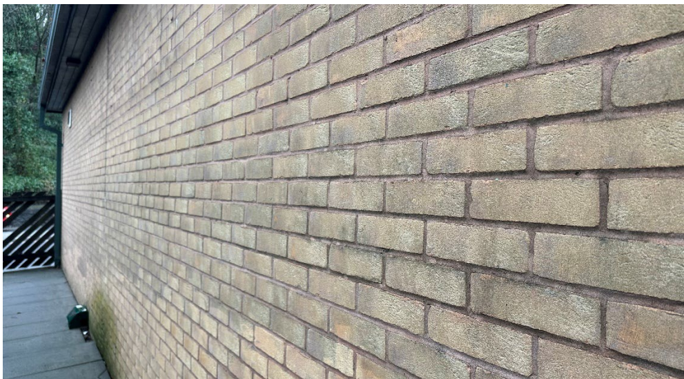
Photo 5: The sales building brickwork is in good condition with no apparent crevices.
