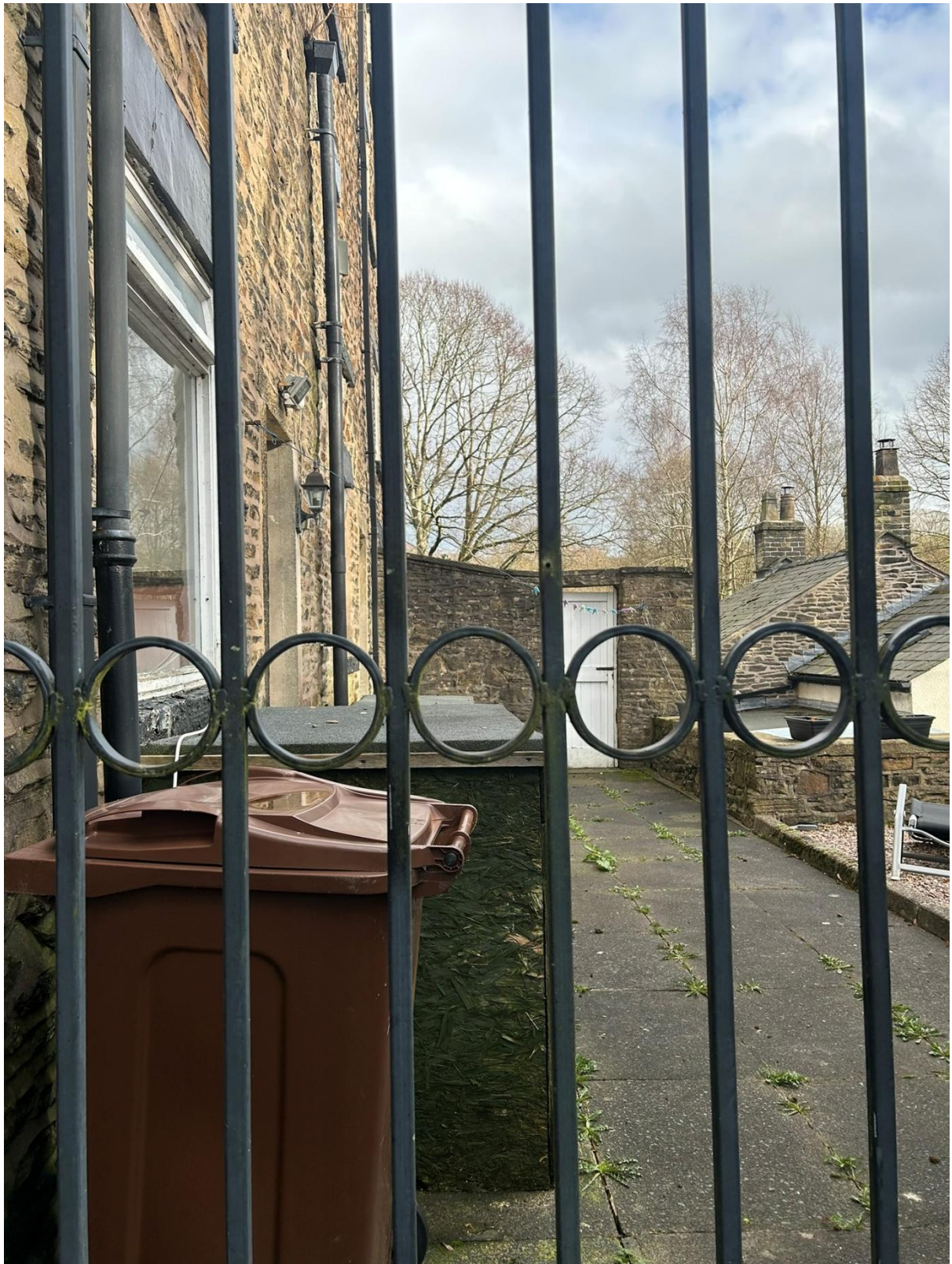
Figure 4: Rear terrace access to No.5 & No.7 and garden area.
