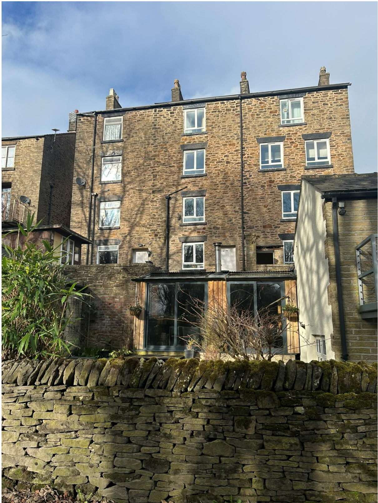
Figure 2: Rear elevation of building showing No. 5 & 7 Riverside. Property in the foreground is a separate residential unit.
