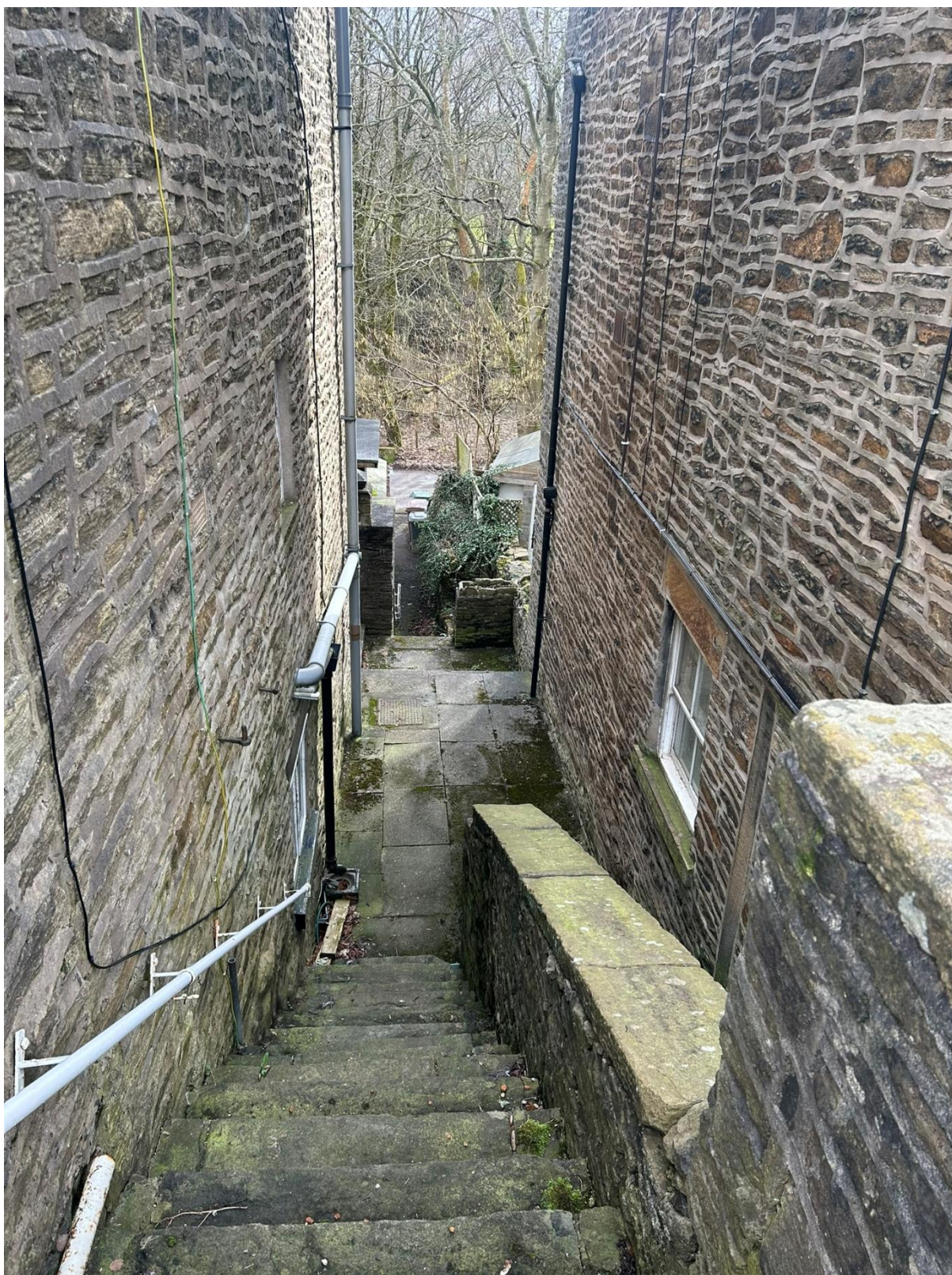
Figure 3: Access to No.5 & 7 Riverside
