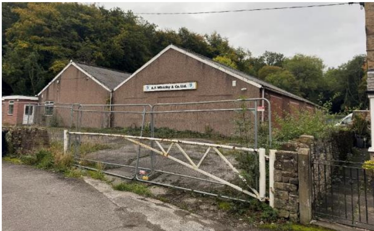
Existing works building to be demolished
