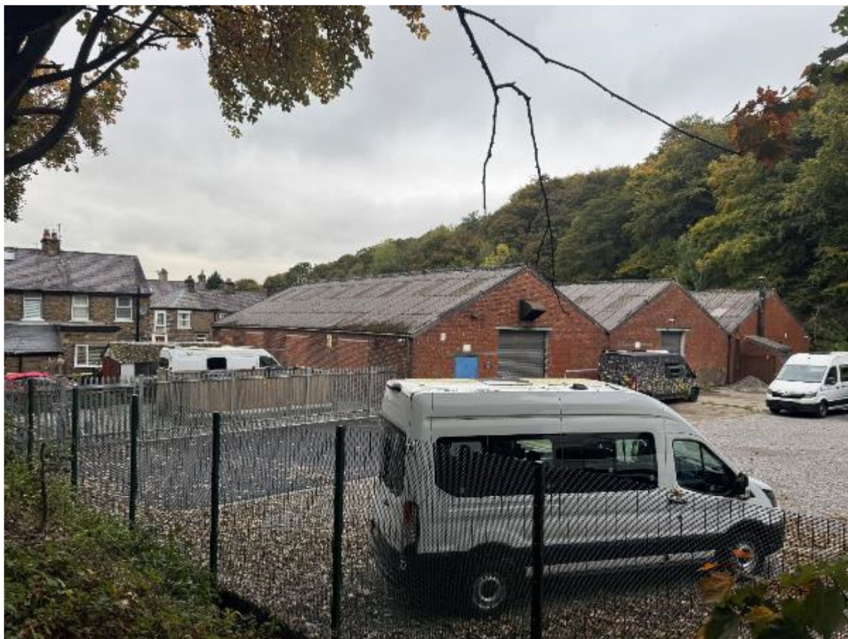
View of rear of existing works building from public footpath to south west
