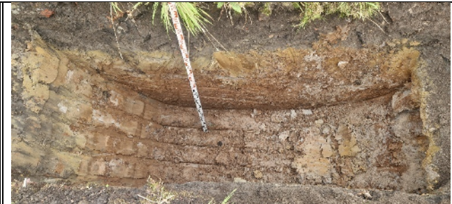
SA01: Internal view of excavation
