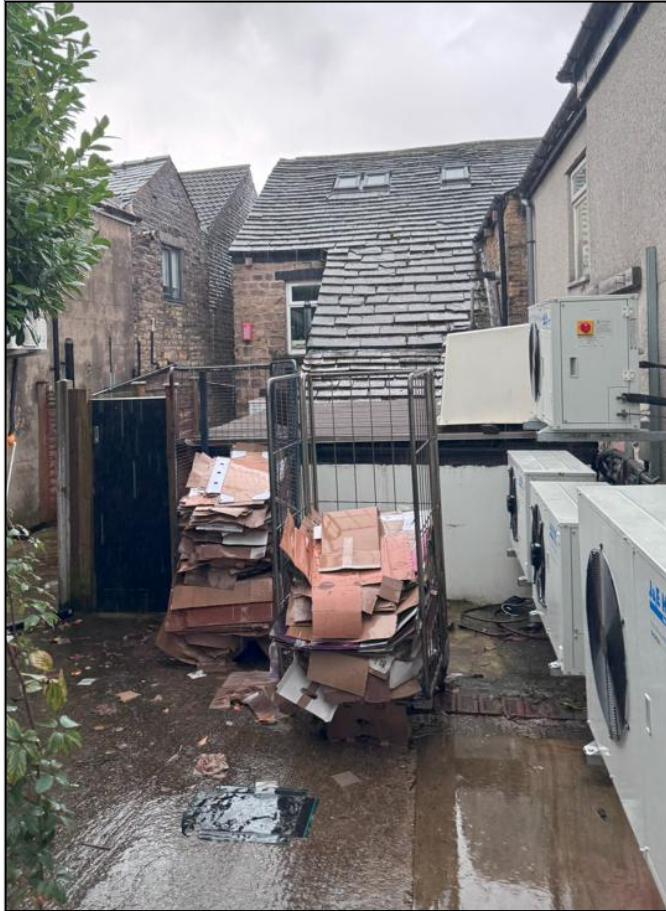
Figure 3: Part Rear (North) Elevation showing the existing cold store
