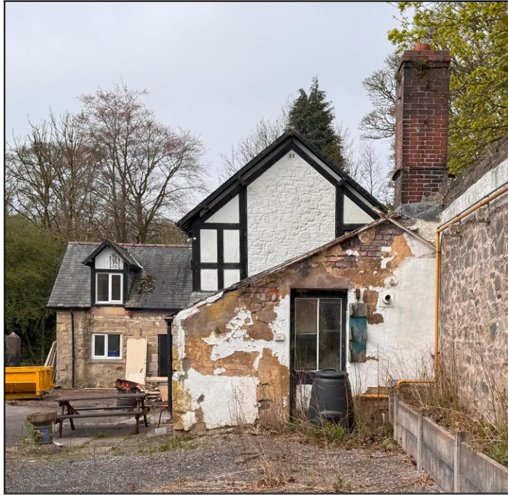
Figure 2: Northeast elevation of the cottages
