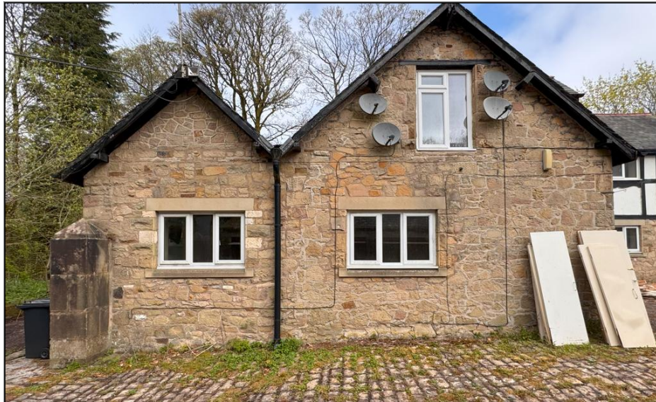
Figure 1: Southeast elevation of the cottages
