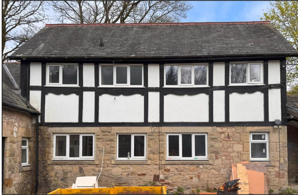
Figure 2: Southeast elevation of the Gardener's cottage
