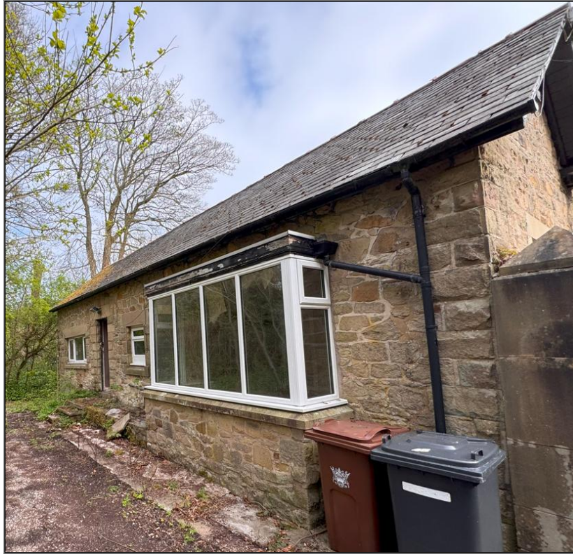
Figure 6: Southwest elevation of the Matron's cottage
