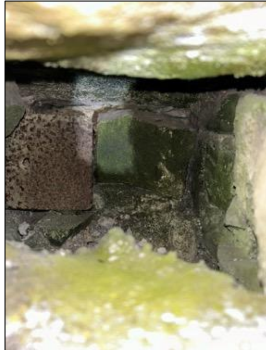
Plate 10. Example of cavity stonework
