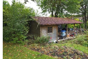
Rear elevation existing garage
