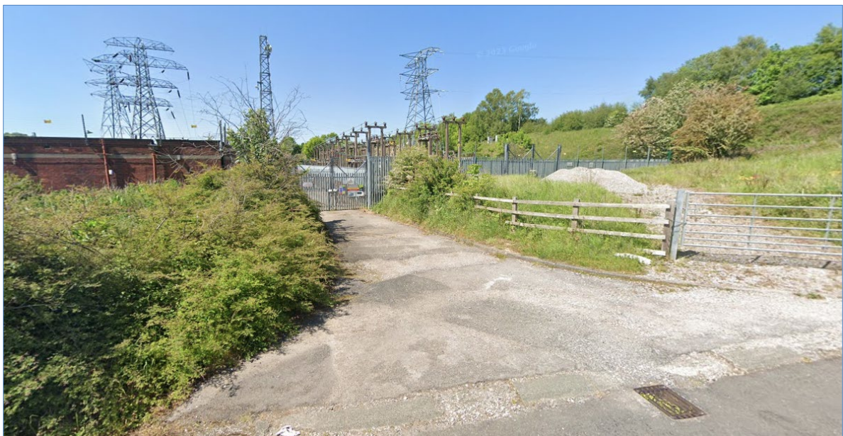
Figure 3: Site entrance at Ladypit Road Electricity Substation where the cable route will end.
