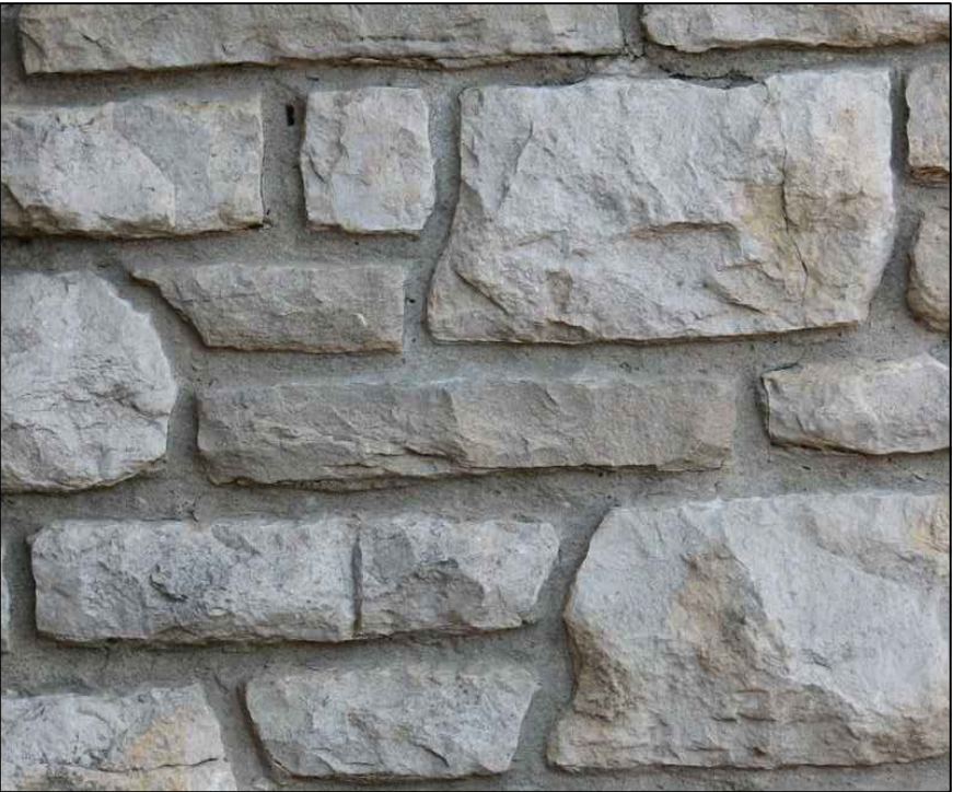
EXAMPLES OF LIME POINTING TO STONE
