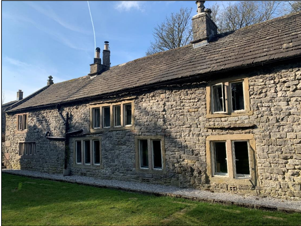
Figure 5 Principal Southern Elevation of Dakin Cottage
