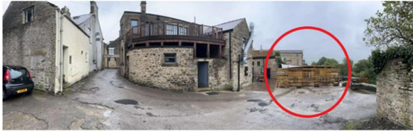
view from rear car park
