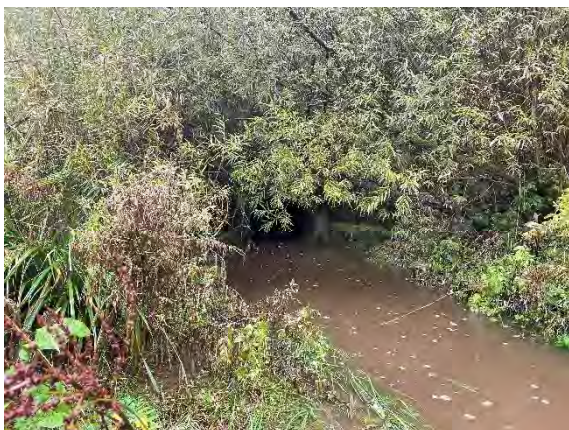
Photograph 16 – Nun Brook, culvert
