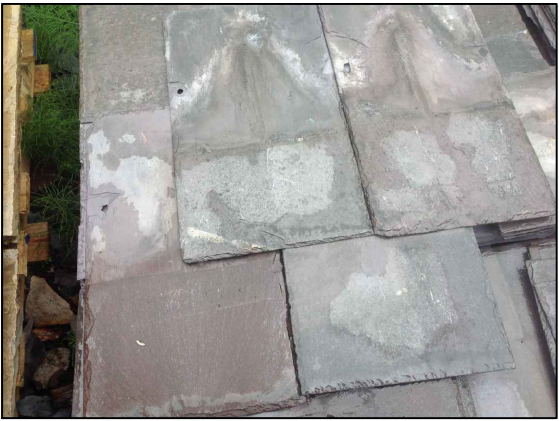
NATURAL SLATE SAMPLE TO NEW BATTEN AND PERMAVENT ROOFING MEMBRANE
