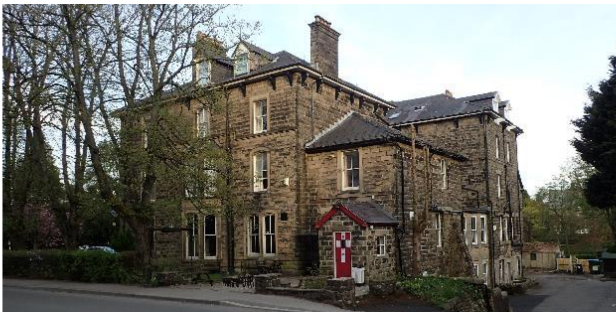
Photograph 2: North and west aspects of Buckingham Hotel, Buxton
