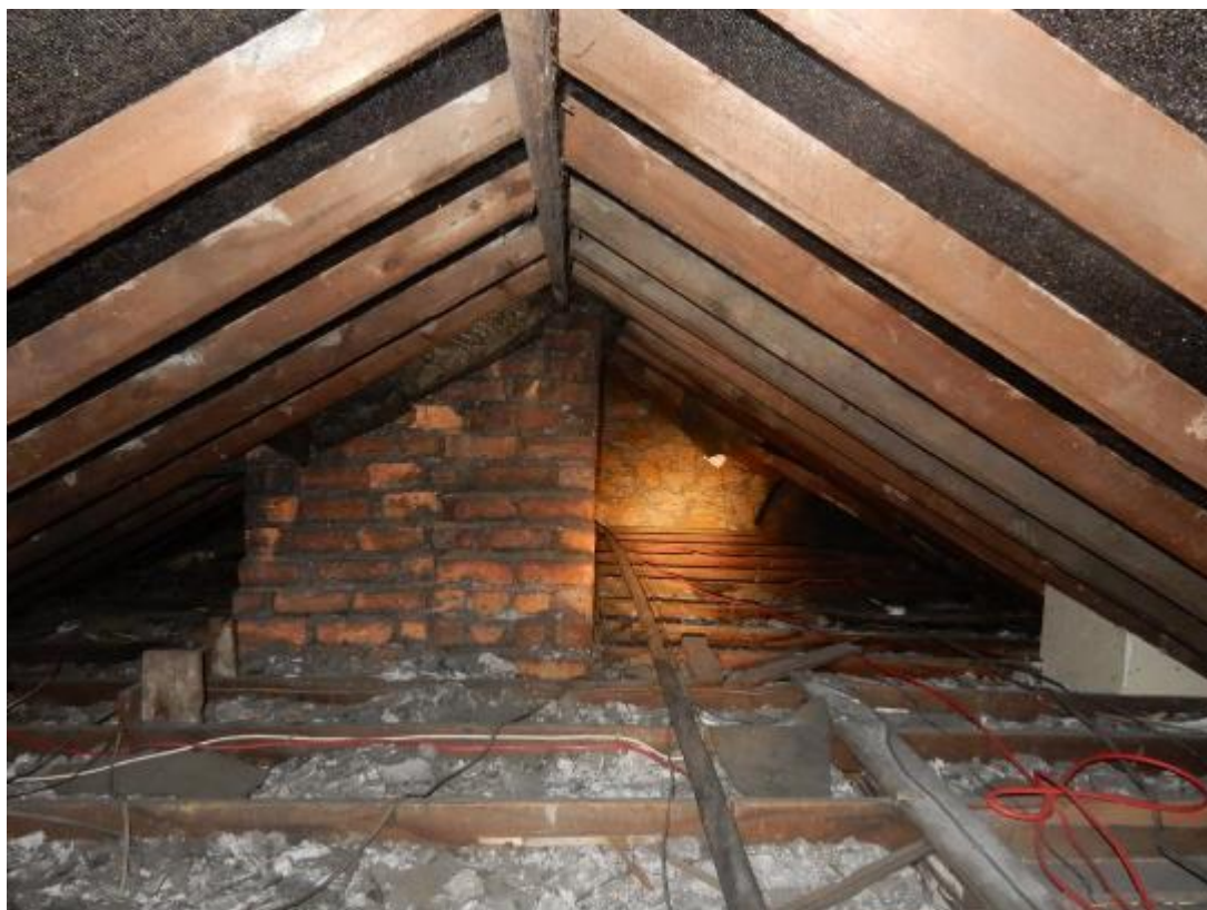
Photograph 3: Typical view of the interior of the attic space over the building
