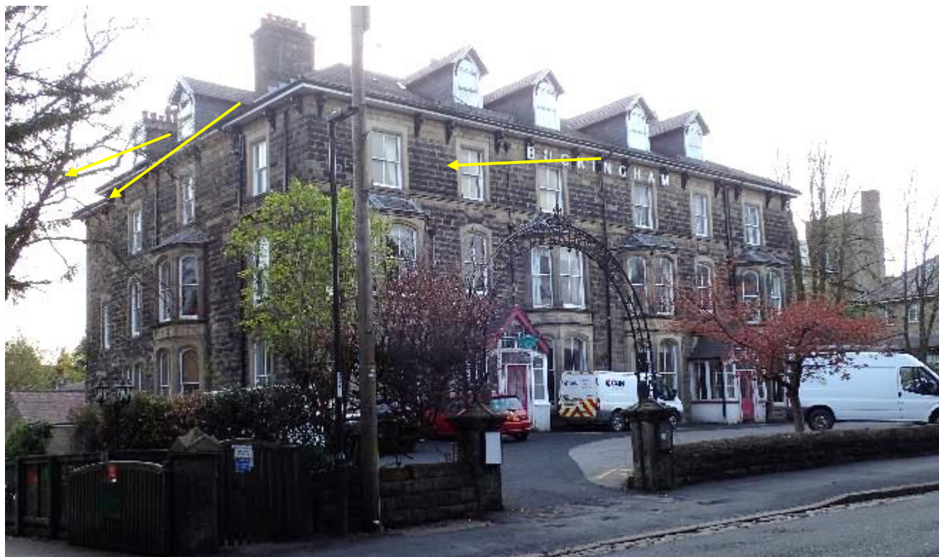
Photograph 7: Annotated photograph of east and south aspects of Buckingham Hotel with emergence points indicated
